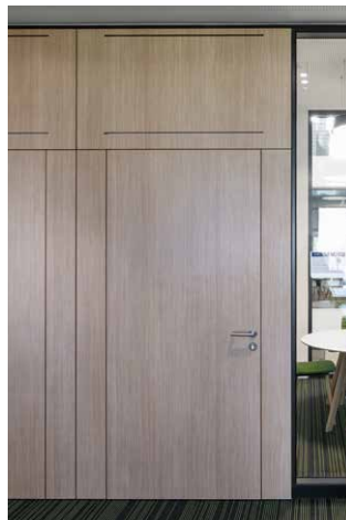
Wooden door element H70 with alum. frame 18/0 and fecoair overflow element
